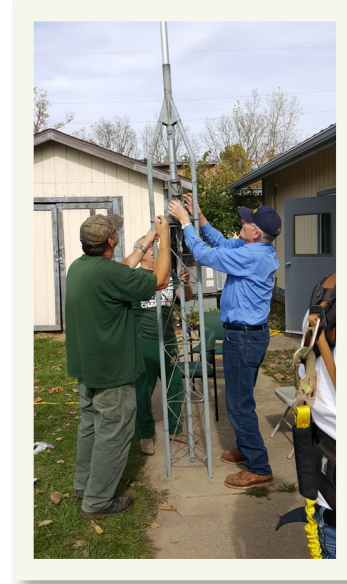
Mark (KD8YUY), Steve (W8RQS), and John (KE8CYC) are adjusting the rotor and rotor plate after inserting the mast pipe which currently holds the dual-band vertical and will hold the Mosley tri-band.
