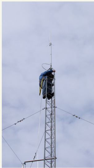
Tom (WA8WPI) on the very top of the tower preparing to raise the gin-pole for raising the Mosley tri-bander.
