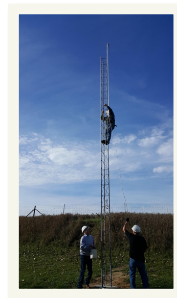
Tom (WA8WPI) adjusting the section tower section and preparing to work his way upward.
