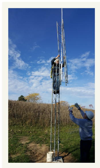
Tom (WA8WPI) on the first section of tower while John (KE8CYC) helps raise the next section via the gin-pole.
