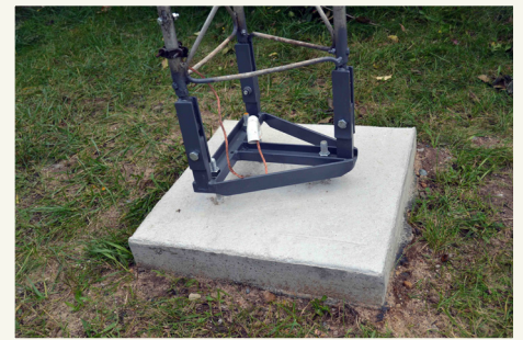
John (KD8NNQ) created a tilt-base for the small tower that once held our 30m vertical. The tower had to be repaired after one of the legs had cracked from ice that had formed inside one of the legs. The tower now holds the short end of our OCF dipole..
