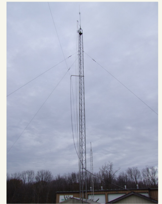
We left the gin-pole attached at the top of the tower waiting for the next day without any wind.
