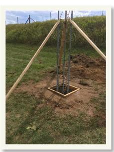
barrel, and then started to backfill. After backfilling, we cleaned up the site, loaded up our tools, and set out for home, waiting for the day we could pour concrete..
