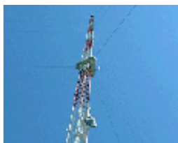
Lansing Civil Defense Repeater Association
