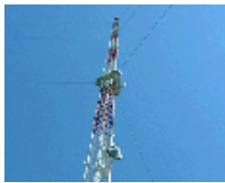
Lansing Civil Defense Repeater Association
