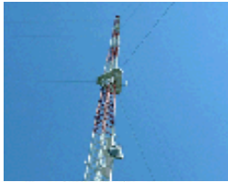
Lansing Civil Defense Repeater Association
