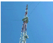
Lansing Civil Defense Repeater Association
