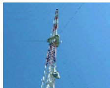
Lansing Civil Defense Repeater Association
