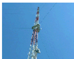
Lansing Civil Defense Repeater Association
