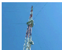
Lansing Civil Defense Repeater Association
